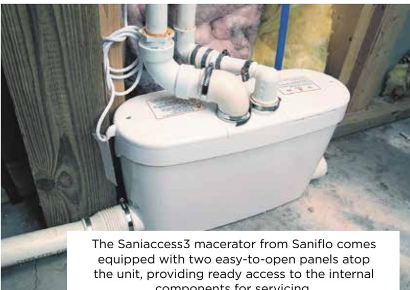
The Saniaccess3 macerator from Saniflo comes equipped with two easy-to-open panels atop the unit, providing ready access to the internal components for servicing.
