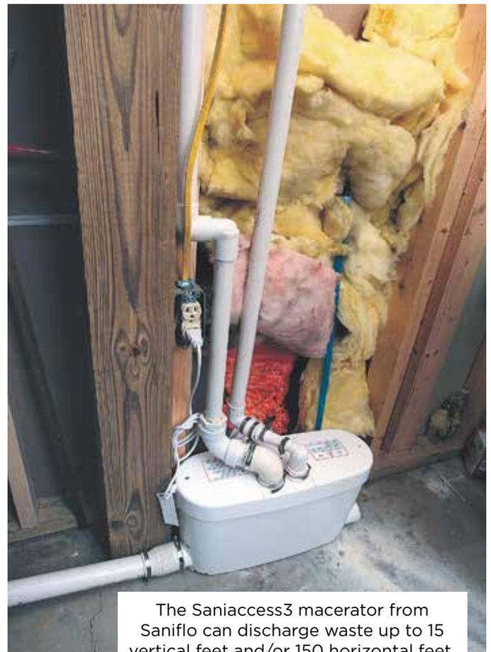
The Saniaccess3 macerator from Saniflo can discharge waste up to 15 vertical feet and/or 150 horizontal feet.
