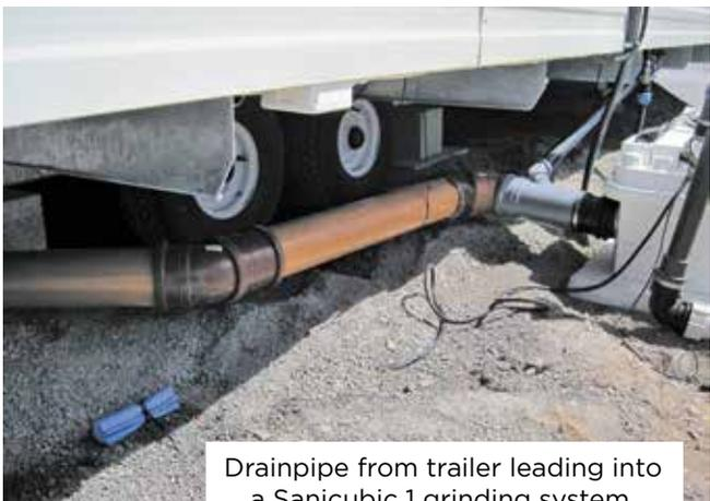
Drainpipe from trailer leading into a Sanicubic 1 grinding system.
